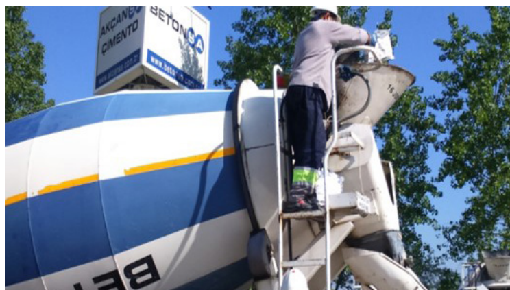
Figure3. High Speed Mixing at least for 7 Minutes
