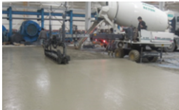
Figure 4. Concrete Placement (with the Laser Screed)
