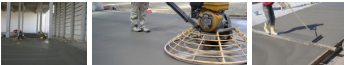
Figure 5. Floor Hardener, Polishing and Brooming
