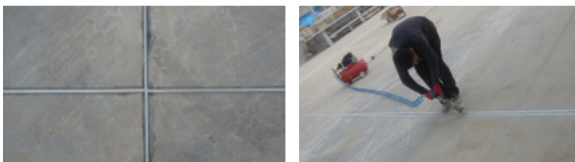
Figure 7. Grouting on Concrete
