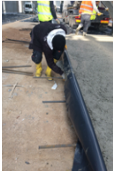
Figure 8. Placing Dowel in Cold Joint Areas
